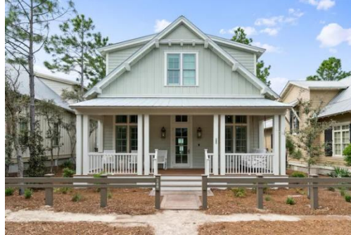
Figure 2 An example of how to emphasize the front entrance to a residence.
